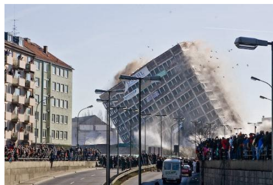
Figure 2. Building demolition using explosives
